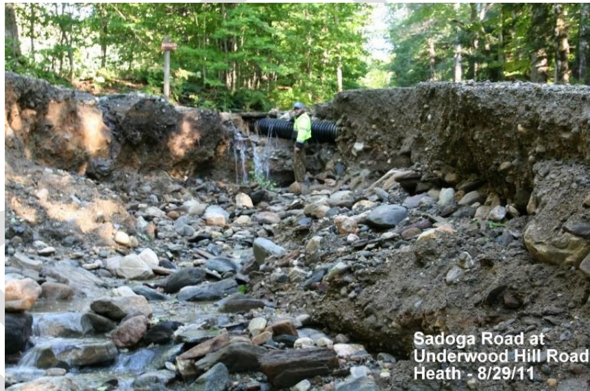
Sadoga Road in Heath was severely damaged by Tropical Storm Irene.
