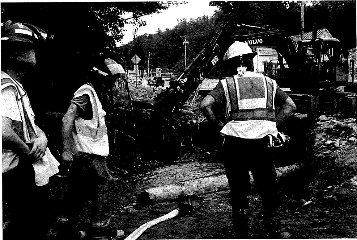
Emergency workers clearing a clogged culvert in Ludlow, Vt., following catastrophic flooding in 2023. Richard Beaven for The New York Times
